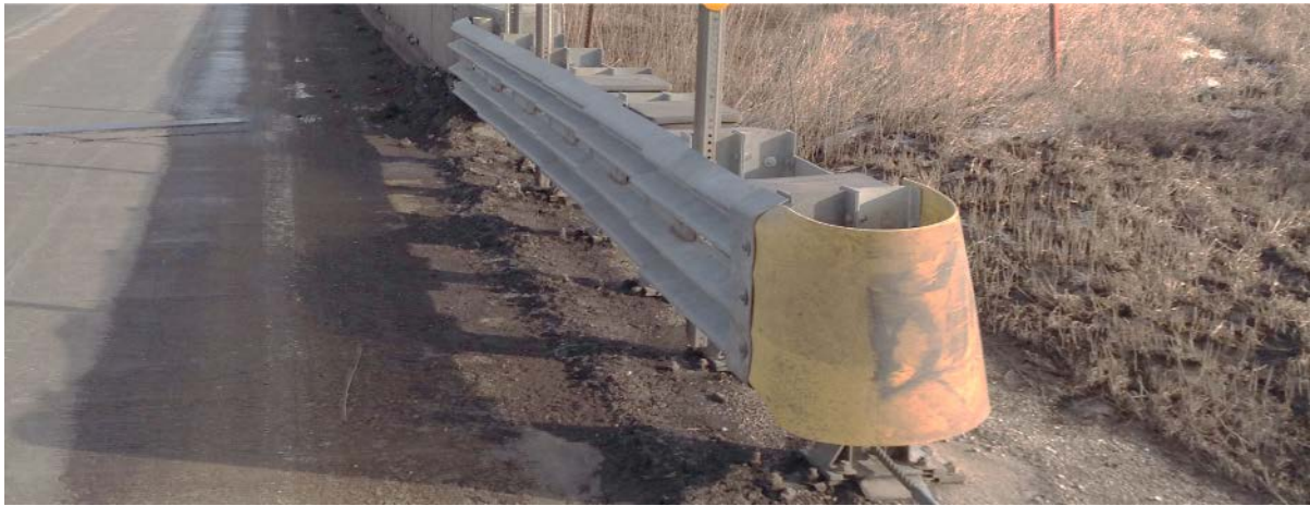
Figure 20. Typical QuadTrend 350 Crash Cushion System (Iowa DOT, 2016)
