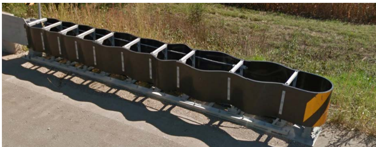
Figure 17. Typical HEART Crash Cushion System (Google, 2016)
