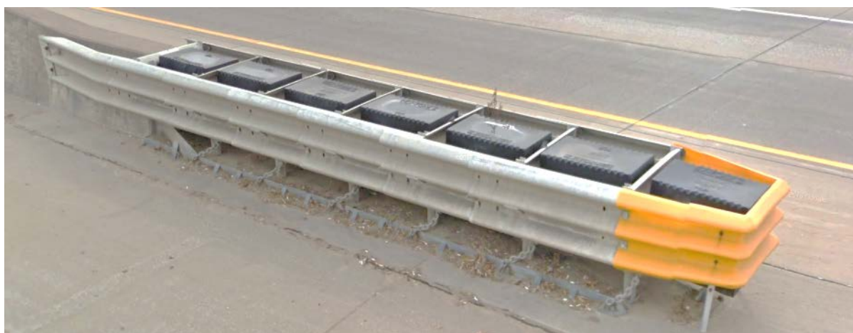
Figure 16. Typical GREAT Crash Cushion System (Google, 2016)
