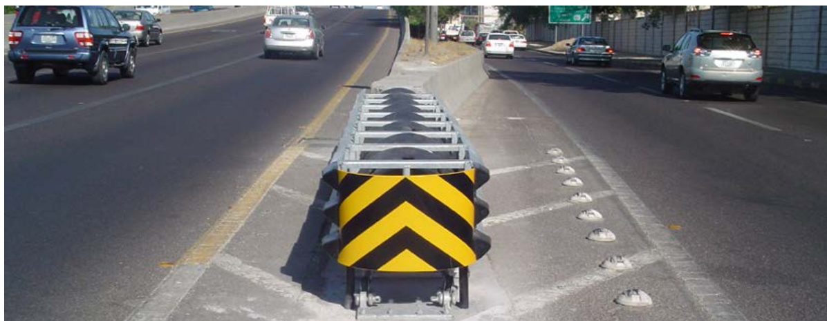
Figure 23. Typical TAU-II Crash Cushion System (Barrier Systems Inc.)
