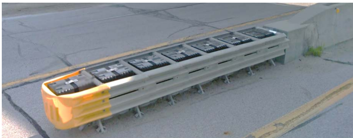
Figure 19. Typical QuadGuard Crash Cushion System (Google, 2016)
