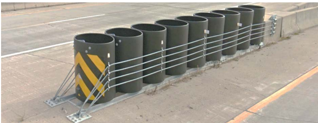
Figure 21. Typical REACT 350 Crash Cushion System (Google, 2016)
